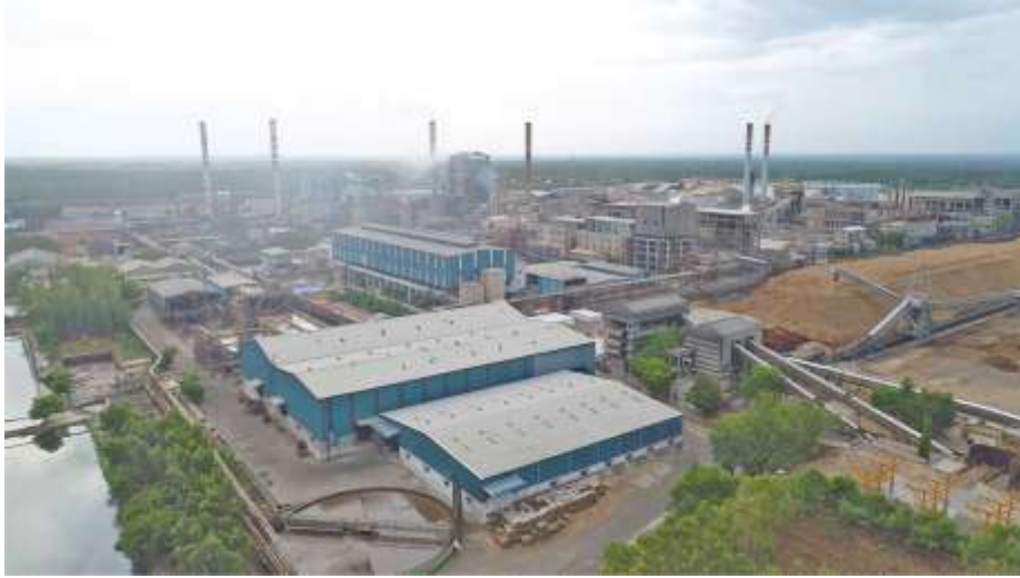
Aerial view of TNPL Unit I facility
