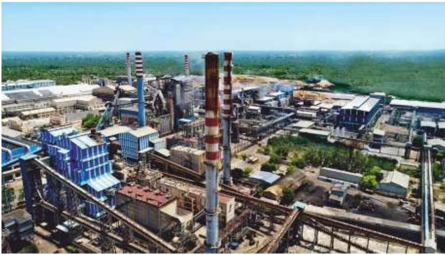
Aerial view of TNPL Unit I facility
