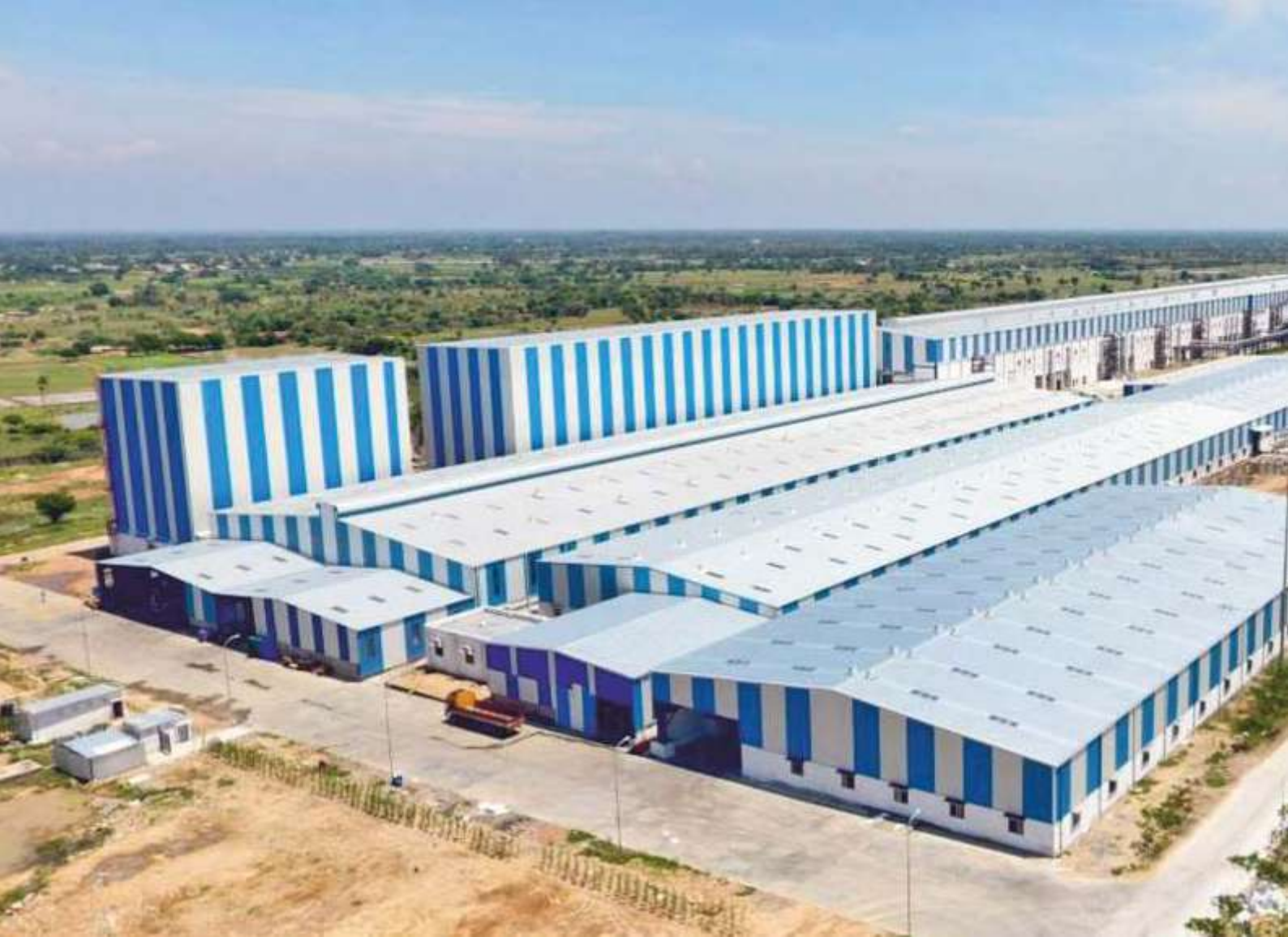
Project Site - Mill Expansion Plan in Unit II under implementation
